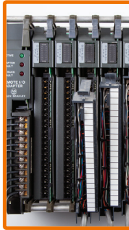
Remove existing Field Wiring adaptors
