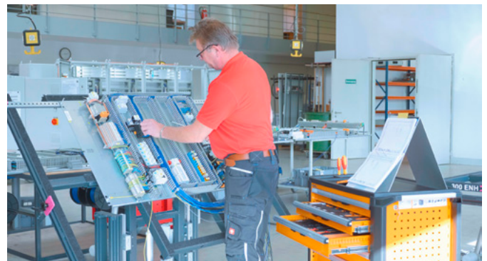
In its modern production facilities, Bosch Building Automation GmbH also insists on excellent quality when selecting surge protection with the VARITECTOR AC range from Weidmüller.
