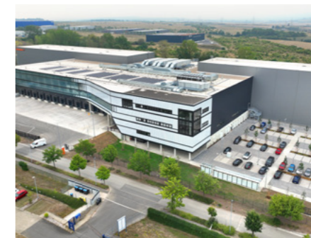
Weidmüller Distribution Center (Logistics Center)
