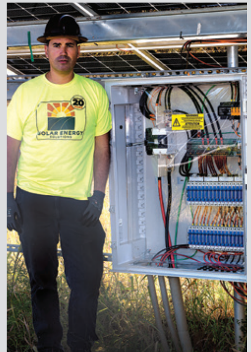
Sized at 1.2 MW DC, Castle & Key's initial solar photovoltaic (PV) is designed to deliver 960 kW AC of clean power to help run its spirits production. A second-phase project is in development to generate an additional 600 kW for the distillery.
