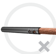
Damaged conductor insulation
